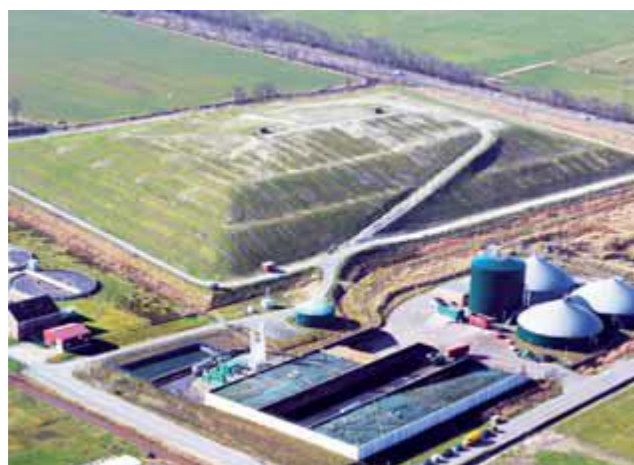
Abbildung 27: Altdeponie in Hage
